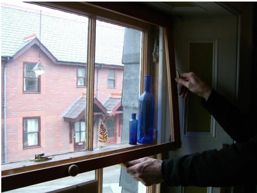
Hinged secondary glazing - bar aligned with original windows for a good match Photo courtesy of www.superhomes.org.uk
